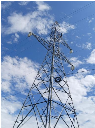
Torres a desmontar
